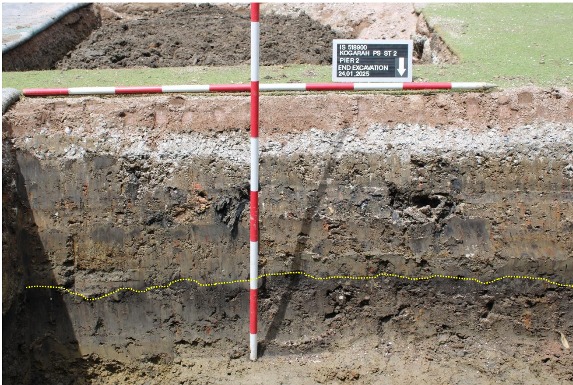
Figure 5-17. Pier 2 end of excavation, example of buried natural soil profile with former topsoil marked with yellow dotted line, facing south
