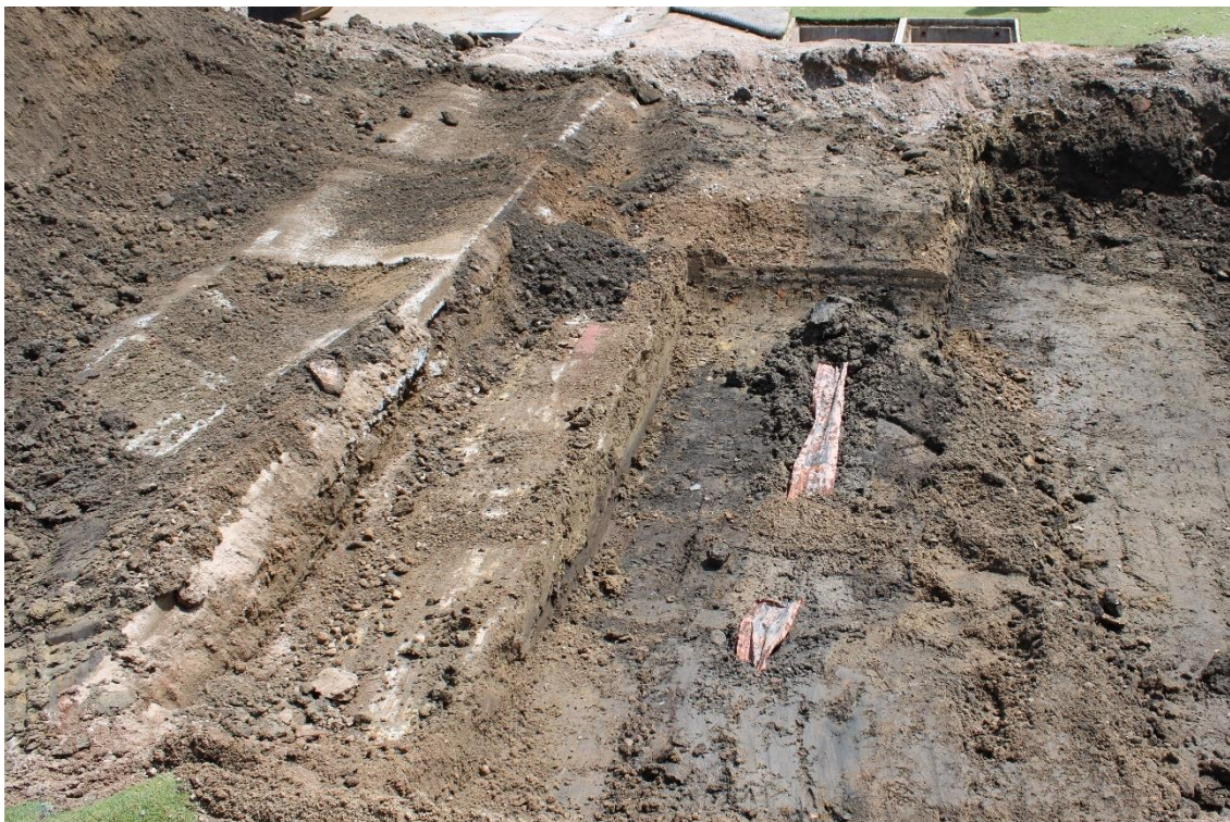
Figure 5-18. Live power utility marked with tape within the bulk earthworks area, facing north
