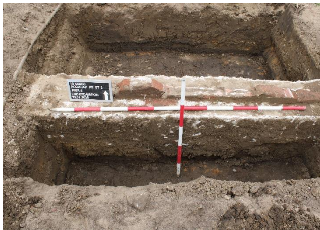
Figure 5-19. Brick and concrete footing, facing north
