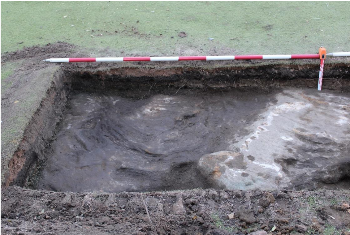
Figure 5-14. Shallow bedrock exposed during in Test Trench Three, facing east
